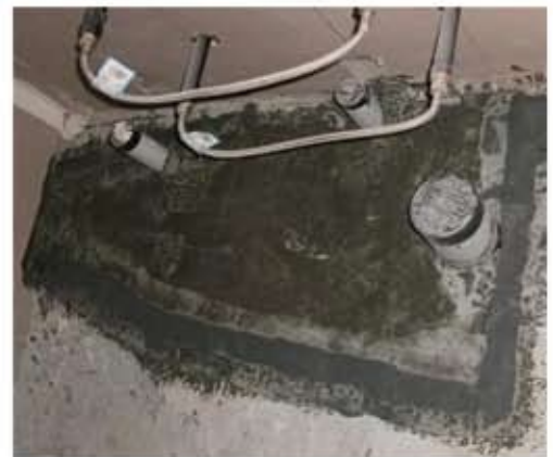
CEMPARGE CONCRETE REPAIR
