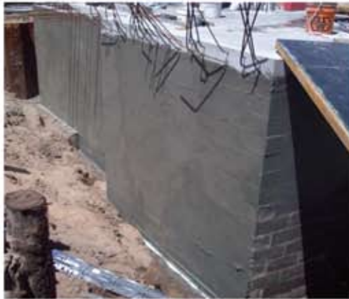
CEMPARGE RETAINING WALL
